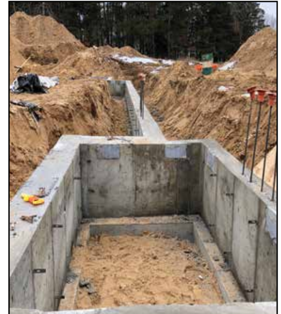
South Wall & Bathroom Footings
