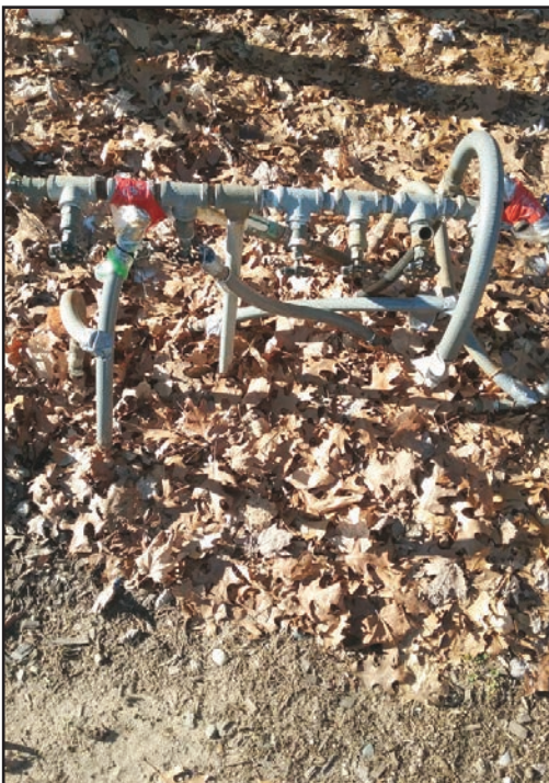
Old Water Riser
