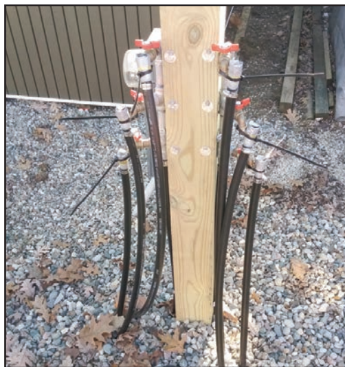
New Water Riser
